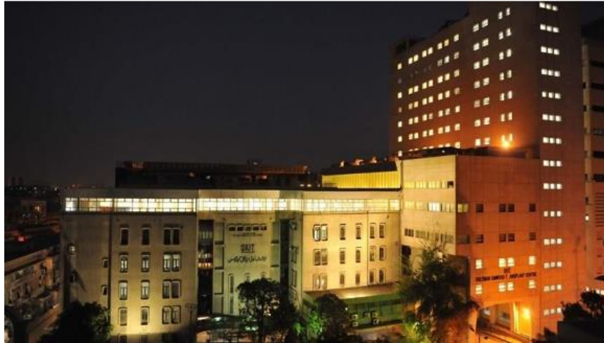
Fig. 2: Part of the SIUT building.
